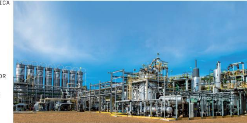
A PLANTA PETROQUÍMICA THE PETROCHEMICAL PLANT
