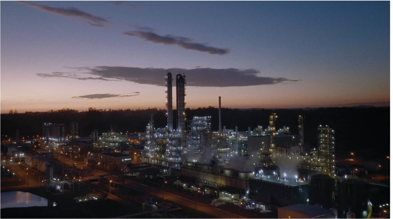
The Steam and Power Generation Plant has 30,000 kW of installed power, equivalent to consumption of a city with 450 thousand inhabitants.
