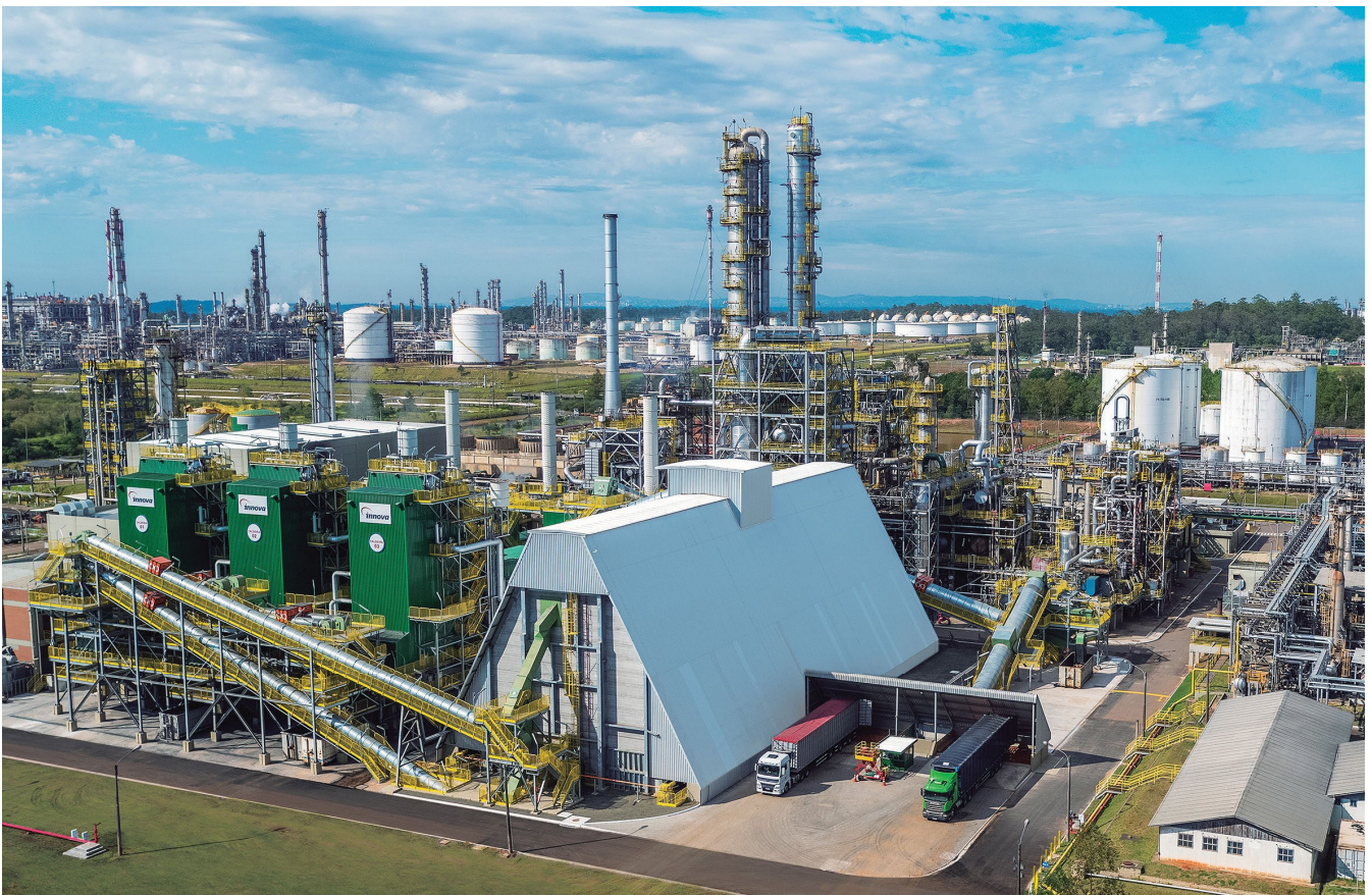
The new energy matrix led Innova to massive neutralization of its greenhouse gas emissions. The Company's commitment is ambitious, heading towards Net Zero in the short term.
