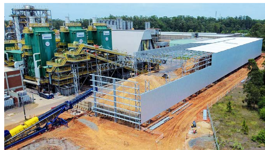
Plant II, Triunfo (Rio Grande do Sul), petrochemical plant: installation of the biomass patio cover.
