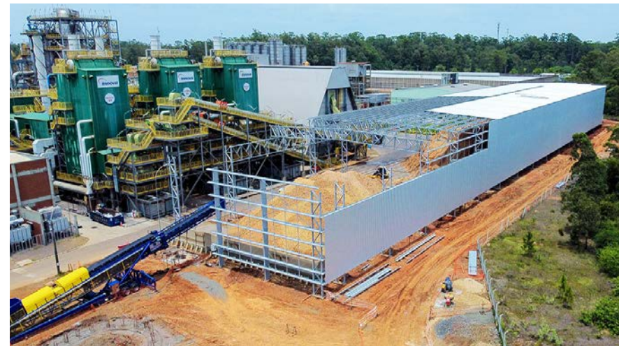
Plant II, Triunfo (Rio Grande do Sul), petrochemical plant: installation of the biomass patio cover.
