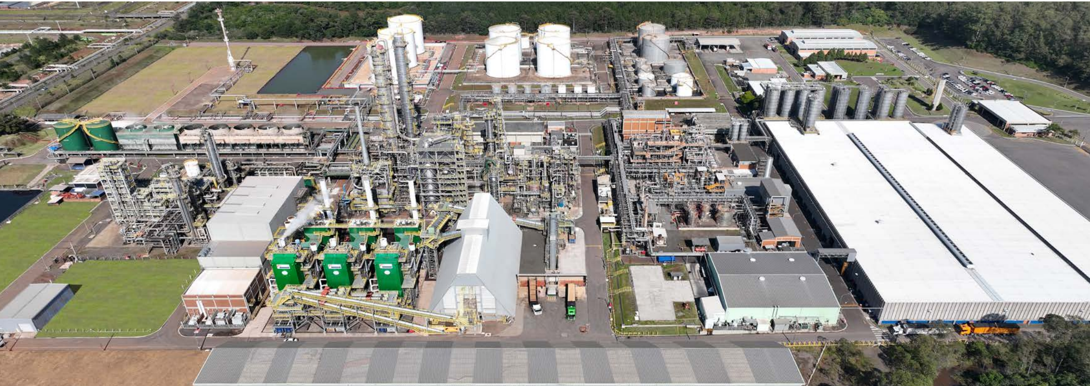
Plant II, Triunfo (Rio Grande do Sul): Steam and Electricity Generation Plant.
